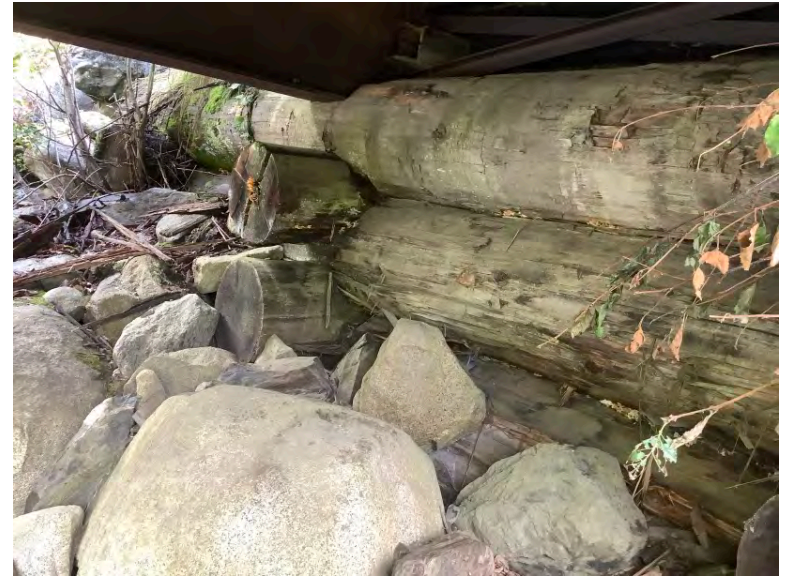
Left Bank Abutment when facing downstream
