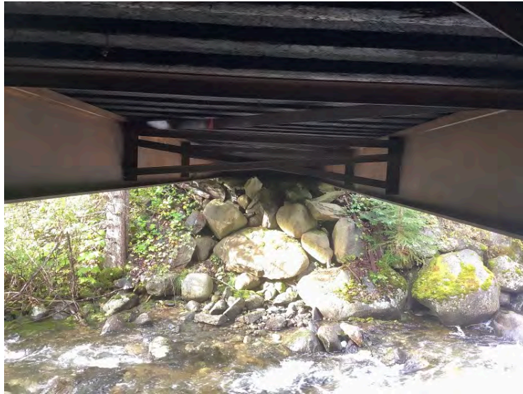
Right Bank Abutment when facing downstream
